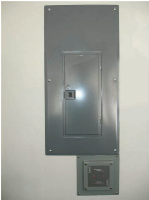
Fig. 7 Sample picture of completely installed unit
